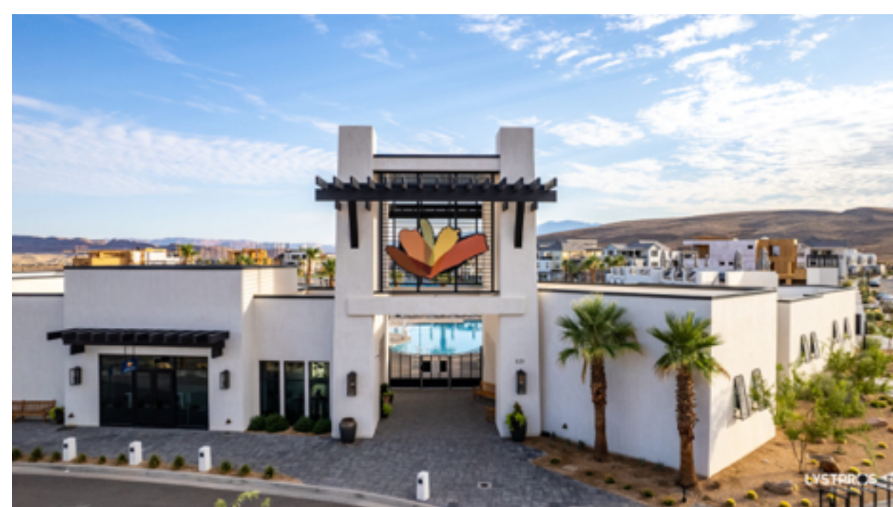
A new master-planned community, is rising just outside St. George. Echoing previous endeavors like Daybreak, Desert Color purports to be a testament to innovation, sustainability and the drive to craft something new amidst the vast desert landscape.
