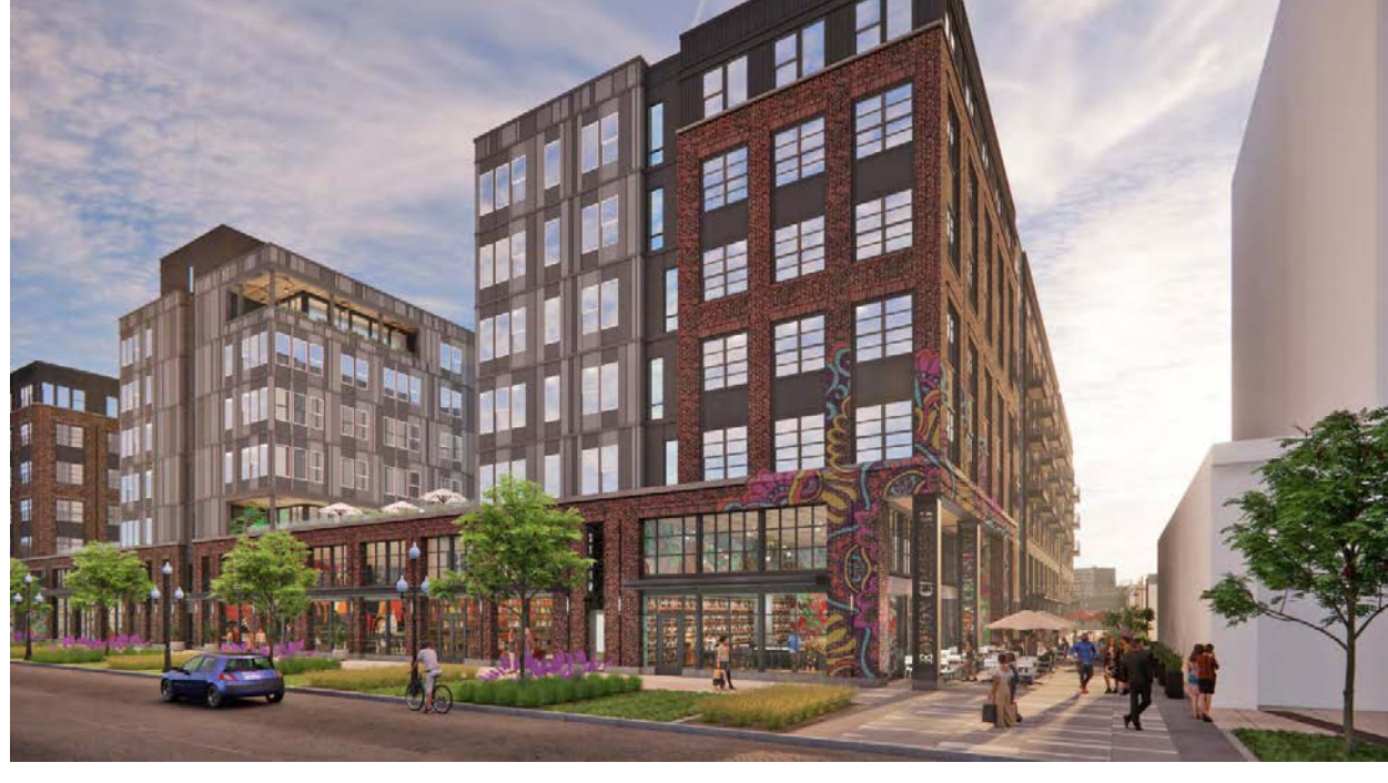
After years of delay and the acquisition of a neighboring property, J. Fisher Companies has rewritten its plans for a significant Downtown site at 250 S. 200 E.
