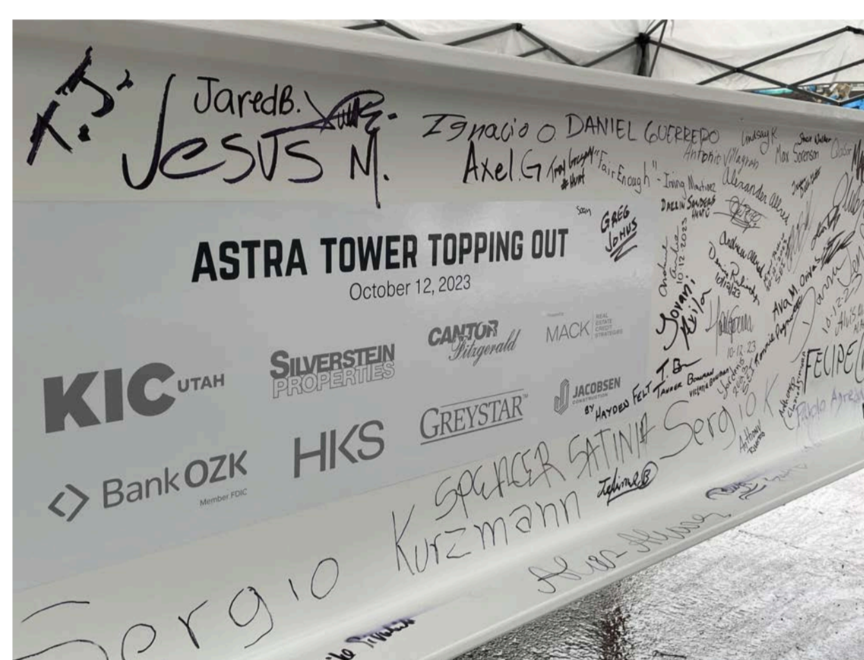
The final steel beam was placed atop what will be a 451-foot high-rise in Salt Lake City, making it the tallest building in Utah. The Astra Tower is located at 89 East 200 South State Street and will house 377 luxury apartments on 41 stories.
