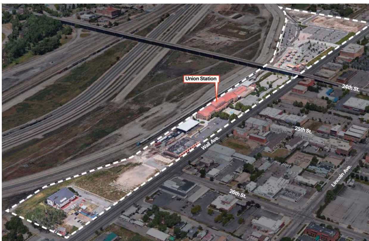
This image shows the area of focus of the Union Station campus redevelopment plans in Ogden.
