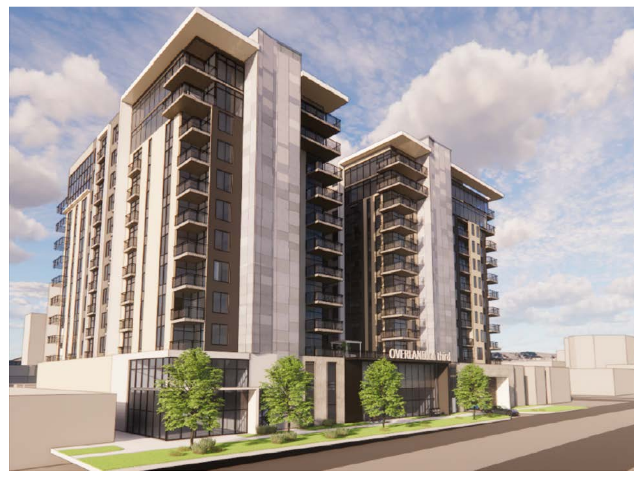
The Overland Development Corporation is proposing Overland On Third, which would create space for 246 residences at 336 South, 300 East
